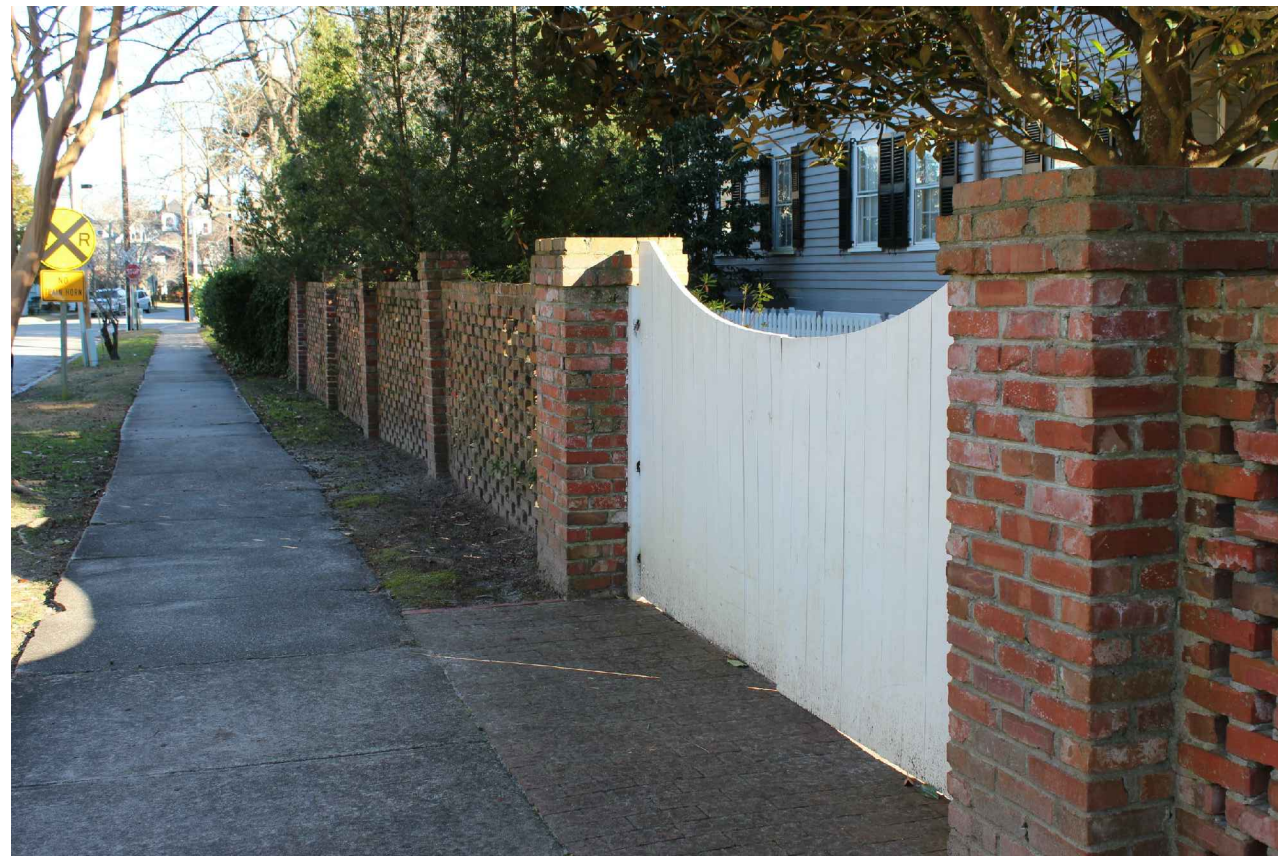
PHOTO OF SOLID PAINTED WOOD GATE ON JOHNSON STREET
