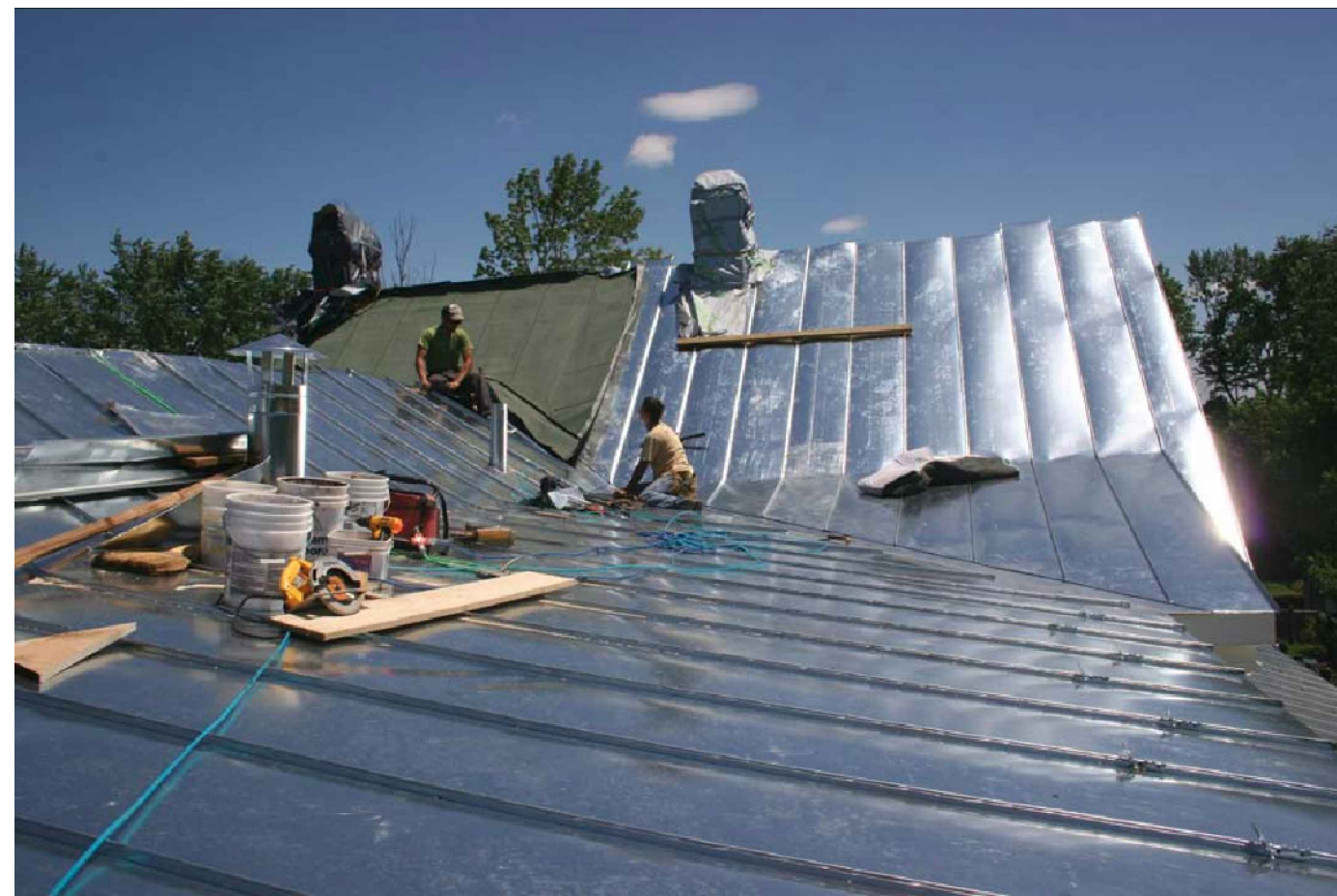
PHOTO OF GALVANIZED HAND SEAMED METAL ROOF
